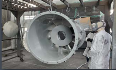
Powder Coating Paint System
