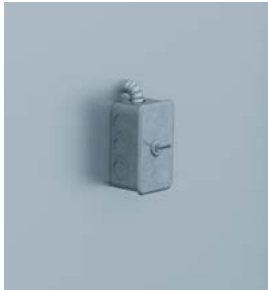
NEMA 1 Disconnect Switch
